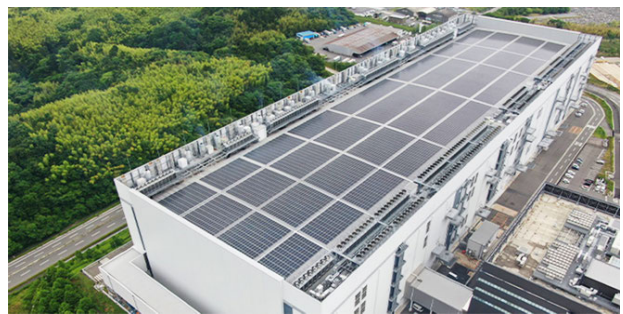
Solar power generation system at Kioxia Corporation's Yokkaichi Plant (Fab 6)
