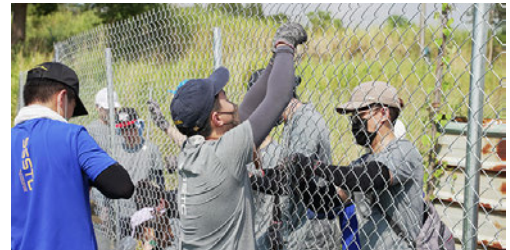
SSSTC employees installing wire netting to prevent Leopard cats from entering poultry farms
