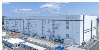
Kitakami Plant (Kioxia Iwate Corporation)
