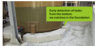
Six-sided inspections Six-sided inspections quickly uncover abnormalities at an early stage
